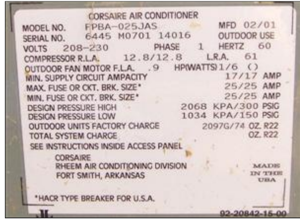
7.8 Picture 2 Data label on compressor.
