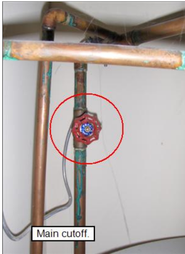
5.3 Picture 1 Lower level closet.
